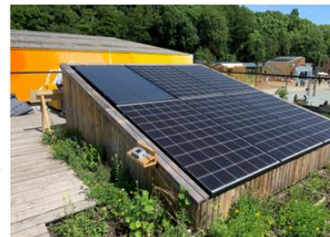
The wood-based building of the VIRTUe team from the Netherlands can be used to add additional floor space to existing buildings. The roof is walkable and includes a PVT field plus a solar collector linked to the house's underfloor heating and cooling system.
