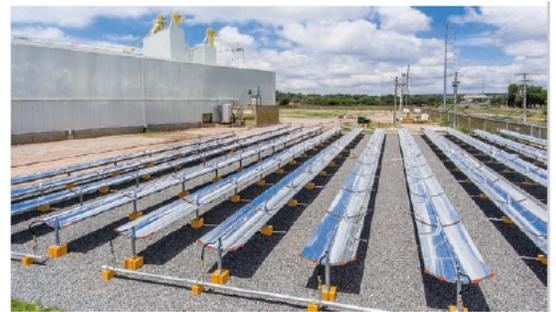
Parabolic trough collectors at Comercial Forrajera de Lagos (COMFOSA) in Mexico. Photo: COMFOSA
