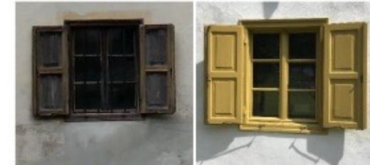
Figure 14: Knablhof (box-type window) – before and after renovation.
