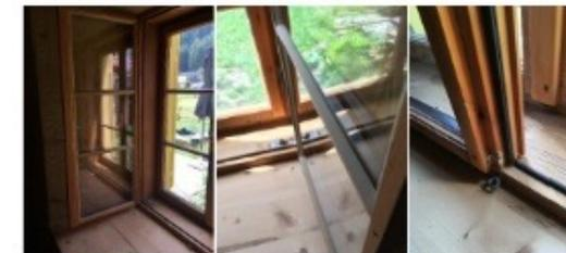
Figure 16: Knablhof (box-type window) – details after renovation.
