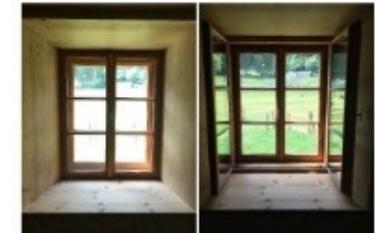
Figure 15: Knablhof (box-type window) – view from inside after renovation.
