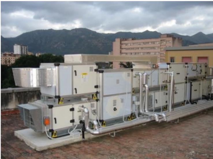
Air handling unit desiccant cooling (AHU-DEC)
