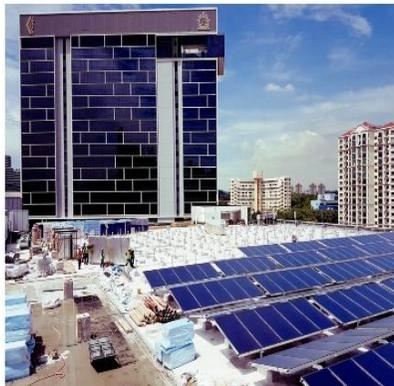
IKEA in Singapore cool is two sales floors, a small office and a warehouse partly with 2,475 m<sup>2</sup> flat plate collectors power 880-kW absorption chiller (250 RT) (February 2018)
