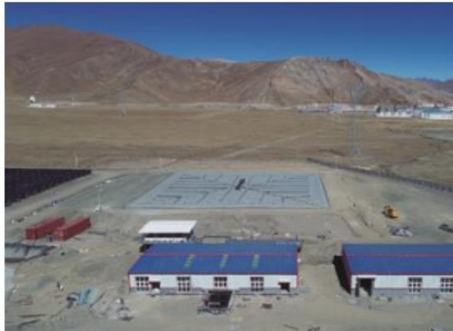
A pit heat storage tank with more than 50,000 m<sup>3</sup> loses 10 to 20 % of the stored energy over the year. The losses depend significantly on the size of the cover.
