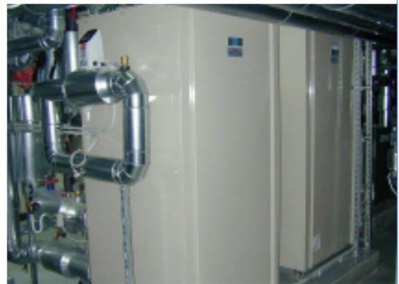
**A solar driven absorption cooling system is used at the German Traffic Ministry in Berlin, Germany. Pictured are the absorption machines (2 x 35 kW<sub>cool</sub>) and the flat plate solar collectors (229 m<sup>2</sup>).**
