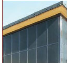
**The Centre d'exploitation des Routes Nationales (CeRN) is a maintenance building of the Swiss motorways. The building is an excellent example of solar thermal collectors integrated into a building façade by adapting an Energie Solaire solar roof system.**
