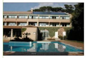
The Golf Hotel in Saint-Raphaël (100 km from Nice) uses solar thermal collectors for their DHW needs and heating the swimming pool. The 90 m<sup>2</sup> of collectors cover 61% of the hotel's hot water demand, saving 37,400 kWh/ year. The collectors also save 20,600 kWh/year in swimming pool heating.
