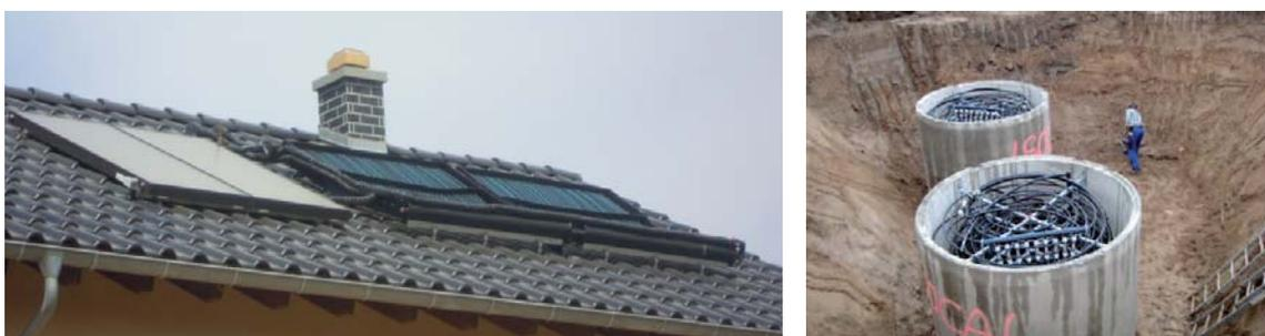
Fig. 3. Solar thermal flat plate collectors (left side of left photo), absorbers (right side of left photo) and ice store (right picture, Source: Isocal)
