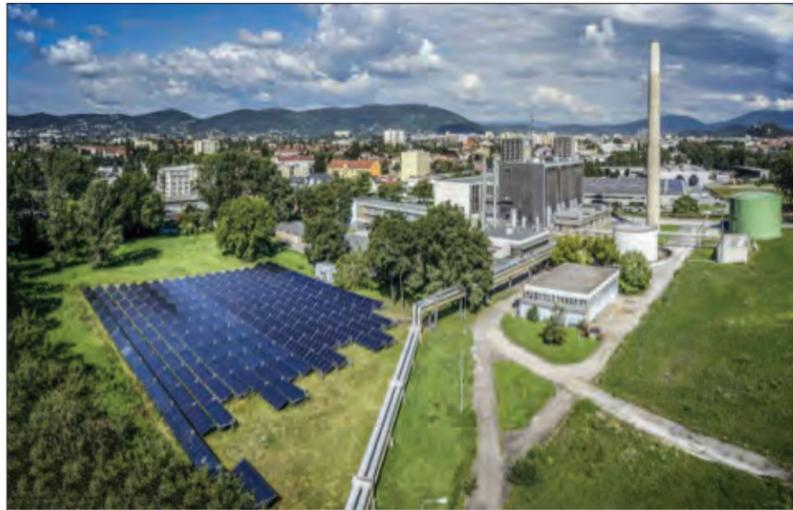
◀ **Fernheizwerk in Graz is the biggest Solar Thermal installation for district heating in Austria.**
