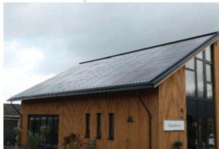
▲ Figure 7. Helios House combines a GB-Sol roof-integrated PV array with a Sunamp compact heat store and a Kensa ground-source heat pump.
