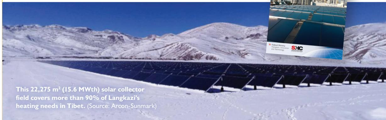
This 22,275 m<sup>2</sup> (15.6 MWth) solar collector field covers more than 90% of Langkazi's heating needs in Tibet. (Source: Arcon-Sunmark)
