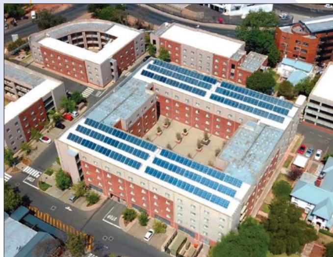
▲ **Figure 4. The WITS Junction solar system is the largest solar thermal installation in Sub-Saharan Africa. The district heating project combines solar, co-generation and gas heating technologies, servicing 14 student residence buildings with hot water from one centralized hot water plant. Installation includes a 600 m<sup>2</sup> solar heating plant with 10 m<sup>2</sup> of collectors.** (Source: Black Dot Energy/SOLTRAIN)
