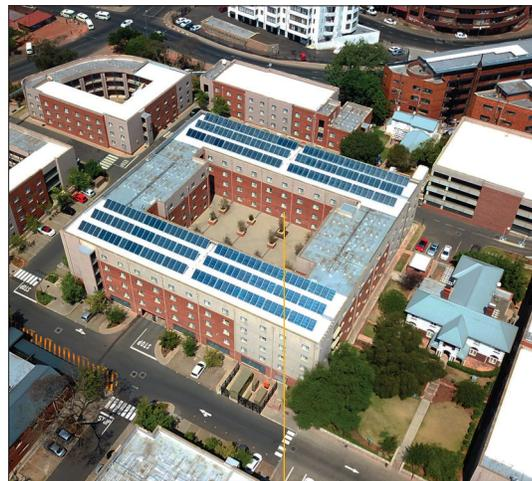
▲ **Figure 1. District heating system on the Wits Junction residence building combines solar thermal, co-generation and gas technologies**
