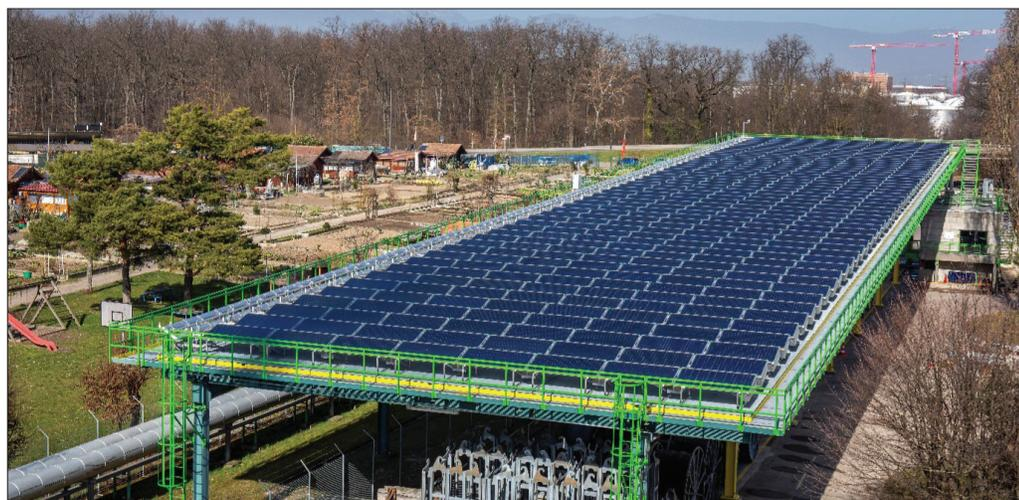
◀ **An 800 m<sup>2</sup> plant with evacuated flat-plate collectors for the return flow boost of the Geneva district heating network. At operating temperatures of 80 - 85 °C, the system achieves an excellent solar yield of 625 kWh/m<sup>2</sup>a.** (Source: Magali Girardin / SIG)
