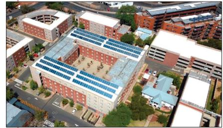
▲ **University of the Witwatersrand Junction Student Residences uses a pumped solar thermal system with a hot water storage tank and external heat exchanger. In one year, this installation gives a solar yield of 397.70 MWh and is responsible for avoiding 137,600 kilograms of CO<sub>2</sub> emissions.** Source: SOLTRAIN
