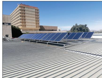
▲ **Thermosiphon systems installed on 58 low-cost housing development in Aussenkehr.**
