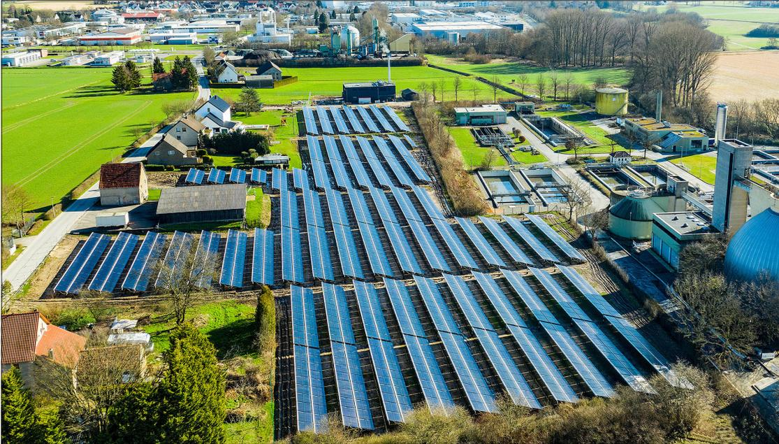
**Solar district heating plant uses 9,181 m<sup>2</sup> of vacuum tube collectors in Lemgo, Germany.** (Photo credit: Stadtwerke Lemgo GmbH/Viessmann)
