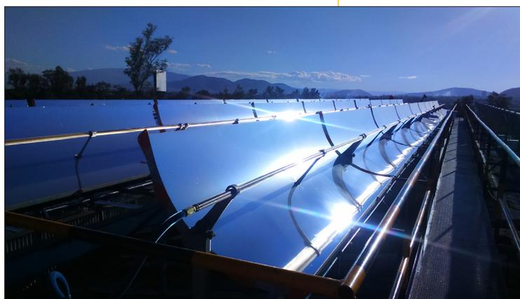
▲ Parabolic troughs used for preheating water at a tequila plant in Guadalajara, Mexico, installed by Inventive Power. (Photo credit: Inventive Power)
