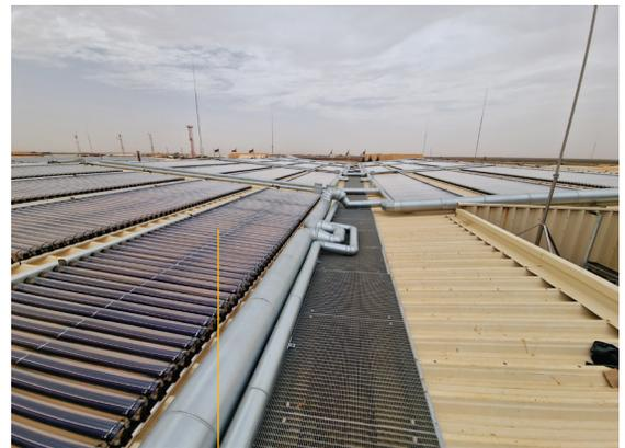
▲ **Solar cooling system at Camp Castor in Mali. The system uses 700 m<sup>2</sup> of vacuum tube solar collectors to drive an absorption chiller with a 348 kW cooling capacity to provide AC to a cafeteria and kitchen. Photo credit: Frank Molter, SolarNext**
