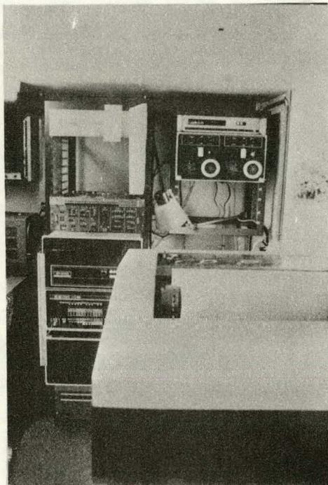
Fig. IV-3. Interior view showing the PDP8/E (for steering the instruments and for primary data processing) and its periphery components: magnetic tape units, line printer and plotter
