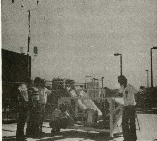
**Fig. III-1:** Preliminary system installation at the Desert Research Institute in Boulder City, Nevada. The majority of system components are mounted on the solar platform - the open frame table in the center of the picture, some of the details of the weather tower can be seen in the left background.
