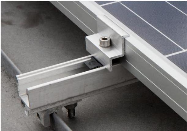
Figure 2 - PV-array on the south-facing roof, reversible mounting by the tin roof fold-clamps, © Pavel Sevela UIBK
