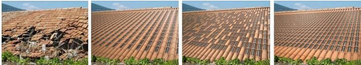
Figure 131: Palmaria Island, study on possible texture of PV curved tiles on a ruined roof
