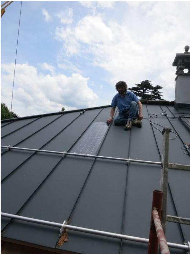
Figure 96: BIPV roof construction, ©Valentina Cari, Progetto Serr@
