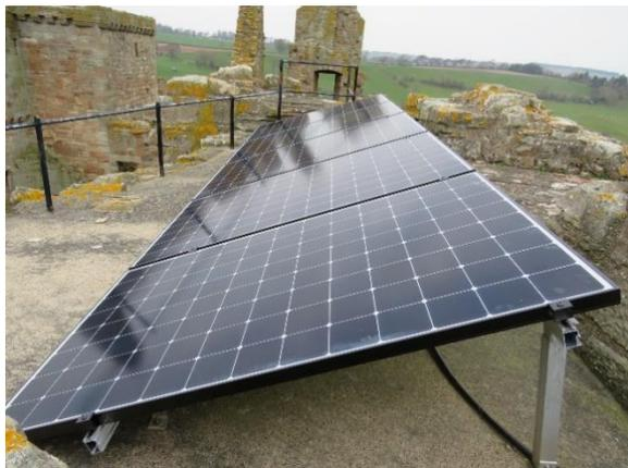
Figure 133: The installed solar panels with ventilation space and incline, © Historic Environment Scotland
