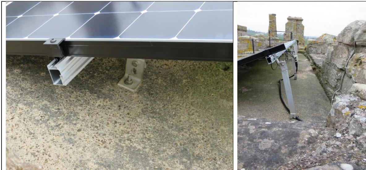
Figure 134: *The fixings into the concrete roof, © Historic Environment Scotland*
