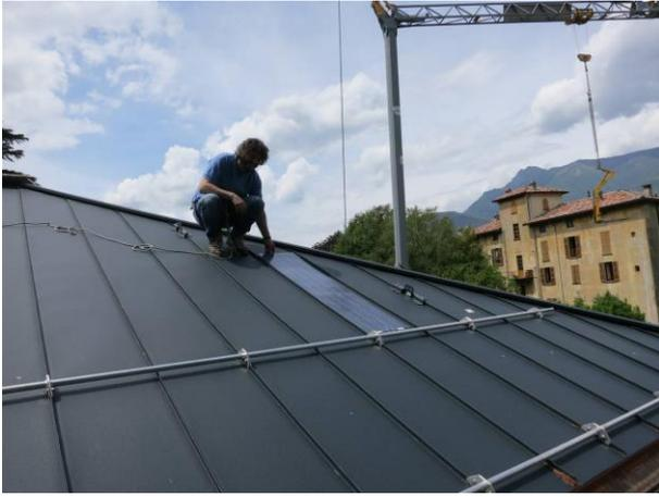
Figure 95: BIPV roof construction, ©Valentina Cari, Progetto Serr@
