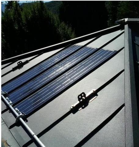
*Figure 140: The PV panel applied on the metal roof,© Valentina Cari Progetto Serr@*
