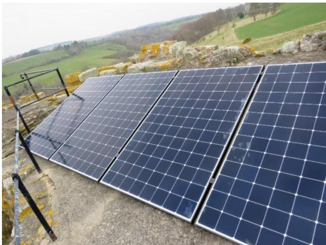
Figure 135: *Incline of the panels to facilitate runoff and self-cleaning, © Historic Environment Scotland*
