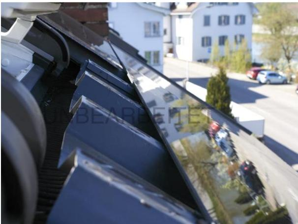
Figure 67: Detail of the solar roof, © Caspar Martig Fotograf GmbH
