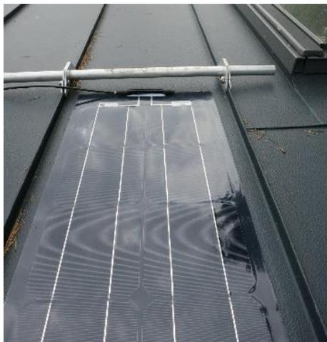
Figure 141: The PV panel applied on the metal roof and connection cables, © Valentina Cari Progetto serr@
