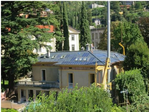
Figure 86: The BIPV roof, ©Valentina Cari Progetto Serr@
