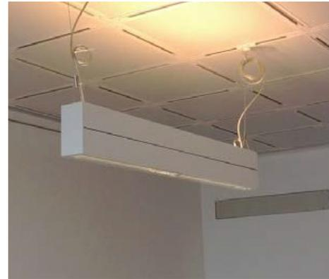
Figure 3. Luminaire with direct and indirect light output.
