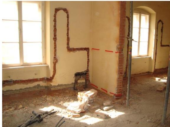
Pipe distribution in the corridor of the monastery for the component low-temperature heating (AEE INTEC)
