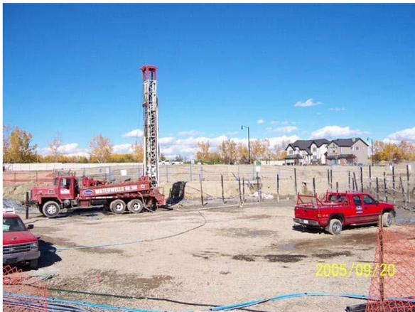
Figure 3. Drilling boreholes
