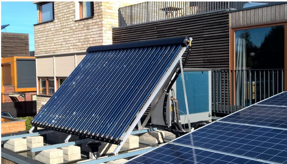
*Conico Direct Solar System combined with air-source heat pump*
