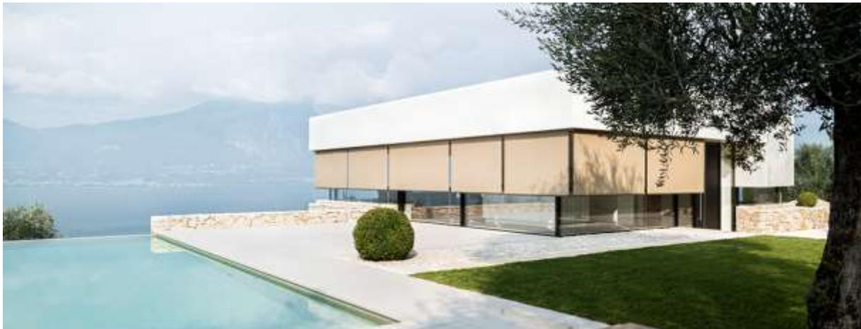
Figure 12. External Textile Shading (Source: <https://www.hella.info>).
