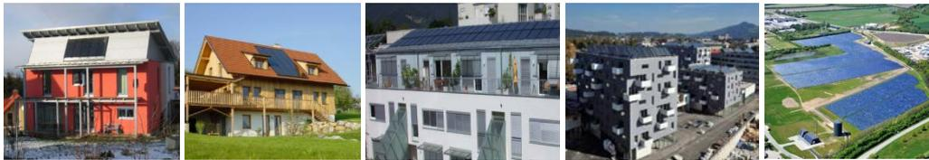
**Figure 3: Typical examples of various solar thermal systems. From left to right, Solar domestic hot water, Solar-combi systems in single family homes, Solar-combi systems in multi-family homes, Solar block heating, Solar district heating.**
