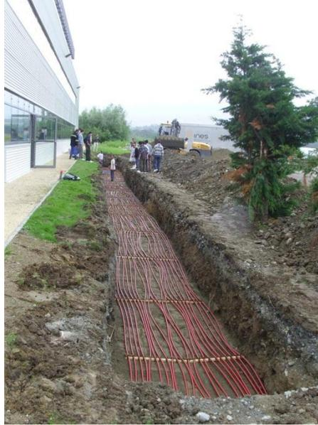
Fig. 10: Example of horizontal ground probe heat rejection system in INES office, Chambéry (source: INES RDI)
