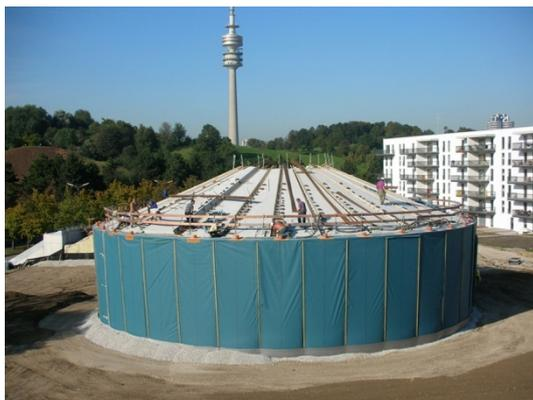
*Filling of membrane casing with expanded glass granules for heat insulation, step by step in combination with outer drainage gravel and earth filling.*
