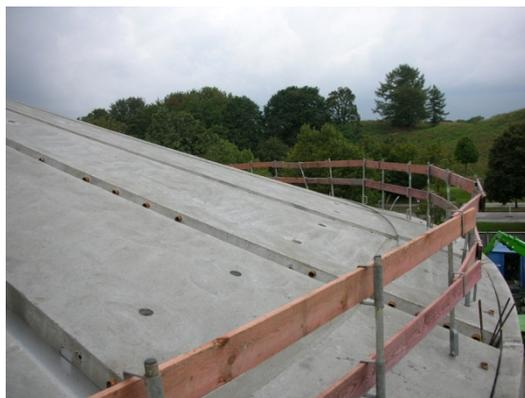
*Mounting of prefabricated roof elements on pressure ring. Inner pre-mounted stainless steel liners for closing of joints*
