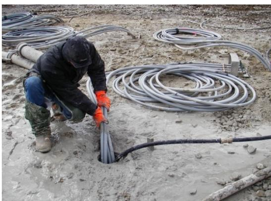
*Filling-up of the upper meters with grouting material. During solification it can occur that the level of the grouting material in the borehole drops some few meters.*
