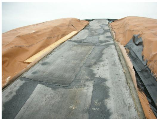
*Mounting of expanded glass granules as heat insulation in geotextile bags in sections on the roof. Each section is finished in one day and closed by a wirtight liner that is open against water vapour diffusion. The liner is glued wirtight against the concrete lid.*
