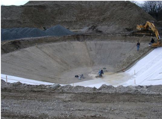
*Emplacement of 20 cm foam glass gravel as lowest heat insulation with geotextile as protection layer*
