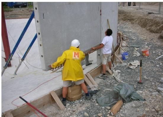
Mounting of first wall elements. Thickness of 16 cm with ductwork for prestressing cables.
