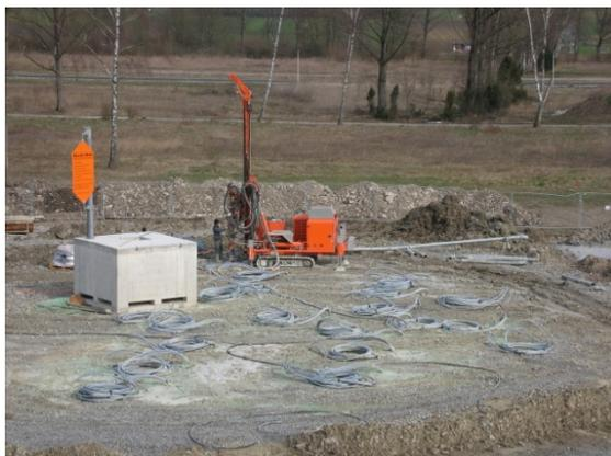
*The boreholes are filled up with heat exchangers and grouting, the horizontal piping is prepared.*
