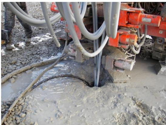
*Filling the borehole with grouting material by pumping it through a hose, the borehole heat exchanger has to be fixed in height until the grouting is solid*
