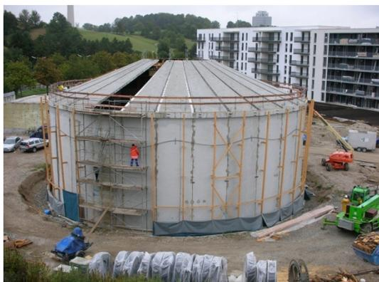
*Closing of the storage lid with two special elements that are located counterpart and integrate the slots for prestressing the lid. Mounting of the outer membrane casing on the wall.*
