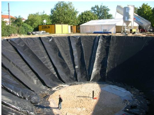
The inner liner is rolled out and welded with some additional liner stripes to large containments.
