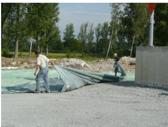
*Always: Protection of heat insulation against rain by covering with foil during non-working time.*
