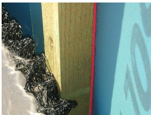
*Cost effective fixing of membrane casing by traditional woodwork, tightening with elastomer layer (red)*
