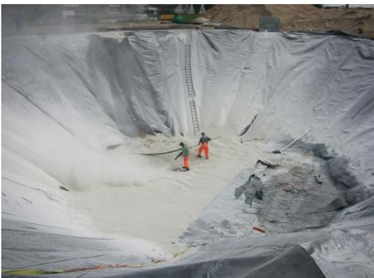
After the inner liner on the walls is welded tight (the tightness has to be checked) the heat insulation of the bottom is blown in. The heat insulation is covered with the inner liner.
