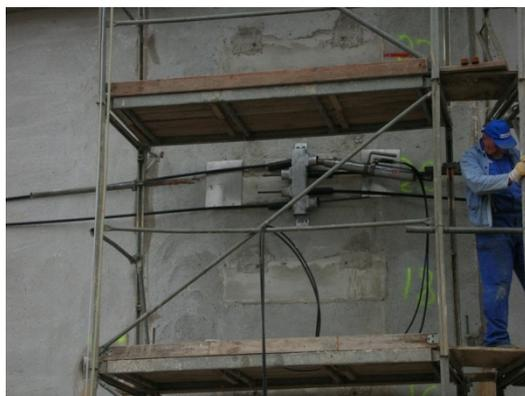
*First time application of high-temperature resisting prestressing cables on outer side of pressure ring.*
