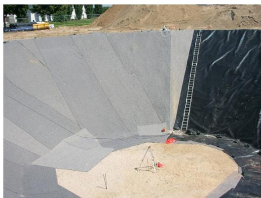
*Laying of the outer liner on inner surface on the protective geotextile. The single lanes of the liner are welded together.*
