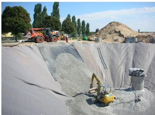
*Filling up of the bottom with gravel to form the lower charging and discharging layer inside the storage.*
