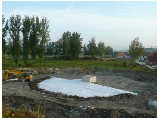
*Covering of gravel layer with geotextile to prevent earth penetrating the gravel layer. On the geotextile earth is filled up.*
