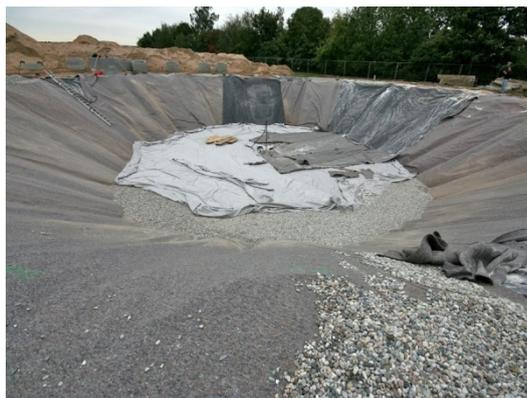
*Separation of the lower gravel layer from the middle sand layer by geotextile that enables water movement and protect the gravel from sand intrusion.*
