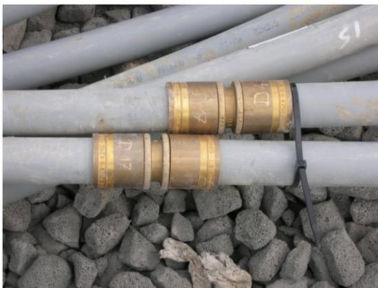
*Pressfittings in detail: the correct connections are labeled by letters and numbers.*
