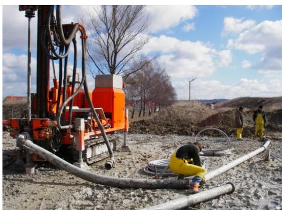
*Drilling works with pumping out of the drilled material through the hose*
