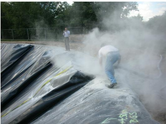
The heat insulation expanded glass granules is blown in the containments via compressed air.
