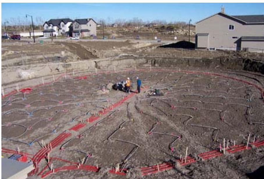
Figure 21: The construction cycle of the BTES in Drake Landing Solar Community (source: Natural Resources Canada)
