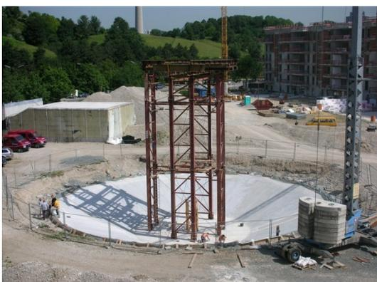
*Concreted lower frustum, in the middle auxiliary construction during mounting of the STES*
