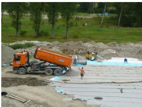
*The covering liners are rolled out. Gravel is dumped on top to build up a drainage layer.*
