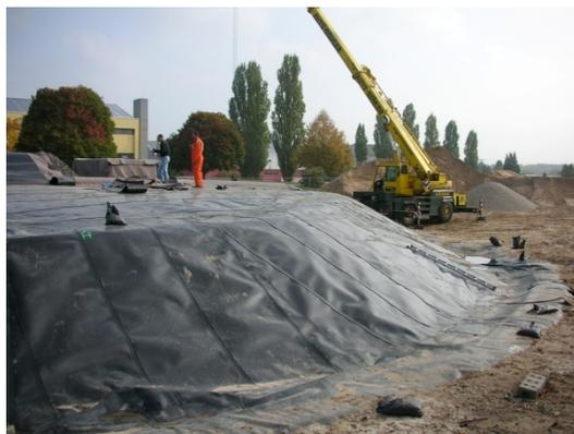
*The roof and slope is coated by the outer liner in lanes and welded together.*
