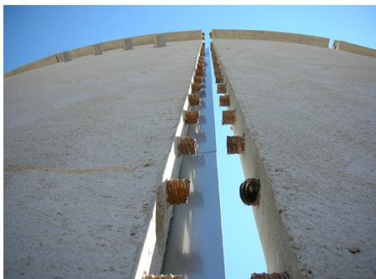
Mounting joint for balancing mounting tolerances (2 times). Inner side with stainless steel liner, 23 ductworks for prestressing over a height of 10 m
