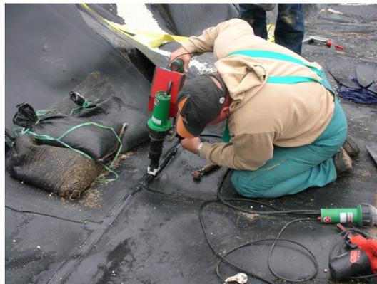
One of the welding methods for plastic liners: manual welding of edges
