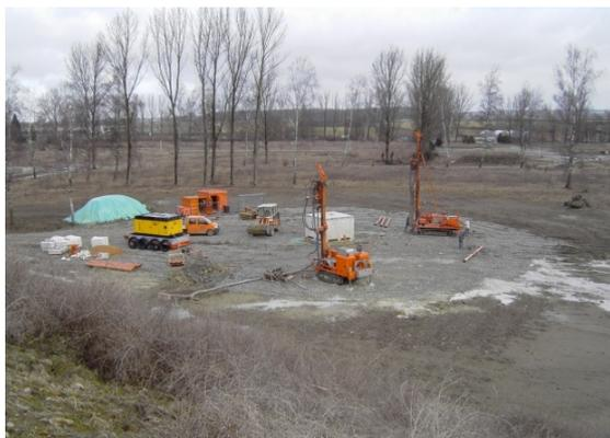
*Second drilling machine works down to 55 m by hammer drilling in the borehole*
