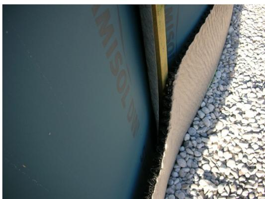
*Protection of membrane casing by geotextile, on the outside drainage gravel*
