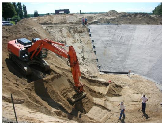
*Leveling of the inner surface of the pit, covering with protection layer (geotextile)*
