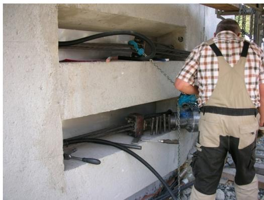
Prestressing of 4 cables in each ductwork by means of a hydraulic press
