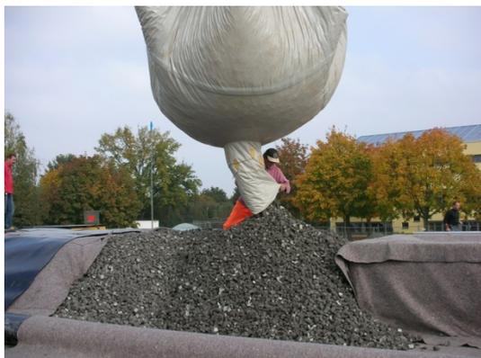
*Purposeful dumping of foam glass gravel with a dumping bag on a crane*
