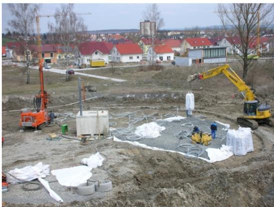
*Drilling work on second storage half and dumping of heat insulation (foam glass gravel) on first storage half.*
