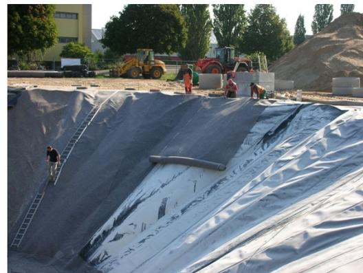
After the inner liner of the bottom is completed, another protection layer is rolled down (geotextile) for gravel-water-pits. For water pits the water can be filled in directly.
