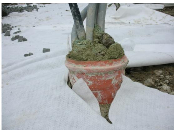
*It has to be secured that the plastic pipes of the heat exchangers are not bended closer than 50 cm. Therefore some of the first protection pipes has to be adapted.*
