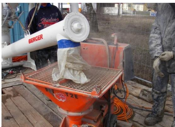
*The grouting material is mixed with water on side. It is highly recommended to use special grouting material that is delivered ready-made on side.*
