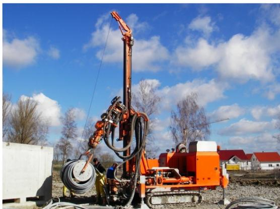
*Rolling in of the borehole heat exchanger from a reel*
