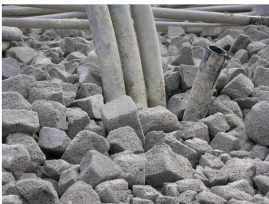
*First layer of foam glass gravel dumped and levelized. The light grey pipes are the borehole heat exchangers, the black one is used for filling in the grouting*
