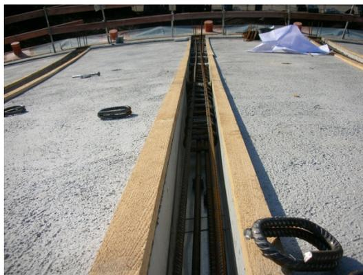
*Closing of the joints on the roof construction by reinforcement and on site concrete.*
