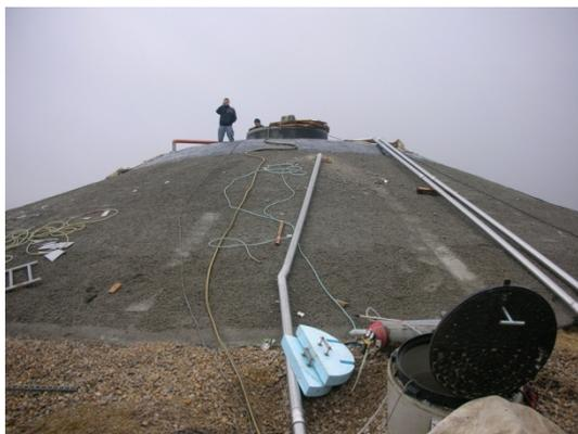
*Emplacement of blinding concrete on watertight liner on the storage lid. Closing of the storage with manhole on top.*
