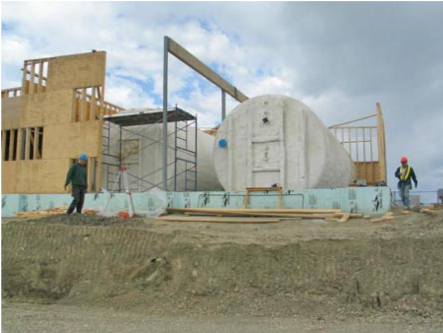
Figure 22: Construction of the heating central with buffer storage at Drake Landing Solar Community (source: Natural Resources Canada)
