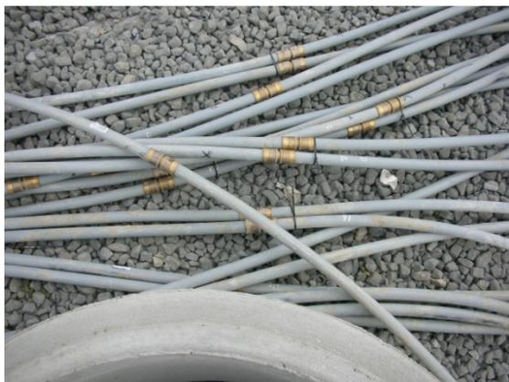
*Roll-out of horizontal piping. Connection of two pipes via hydraulic pressfitting. Due to the crosslinked character of the piping no welding is possible.*
