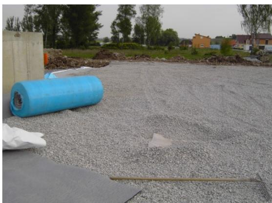
*Heat insulation of horizontal piping by second layer of foam glass gravel. On the left side the central shaft is visible.*
