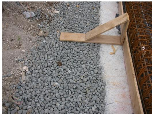
*layer construction on the edge between storage bottom and wall: on the right the wall socket, in the middle blinding concrete, left: foam glass gravel as heat insulation*
