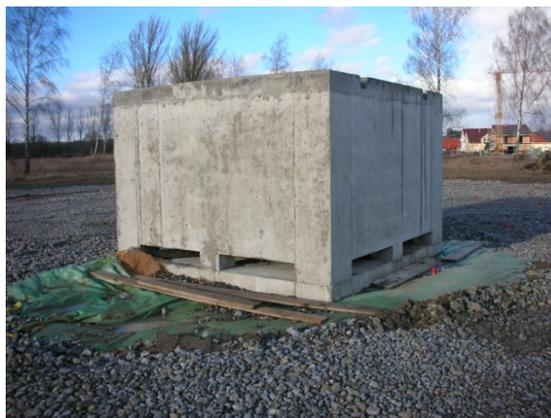
The central shaft for connection of the horizontal piping is put on a layer of heat insulation (foam glass gravel)
