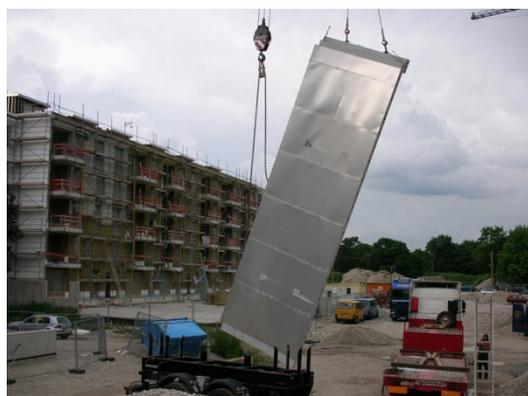
*Delivery of prefabricated concrete wall elements with inner stainless steel liner, welded of 1,2 mm stainless steel plates.*
