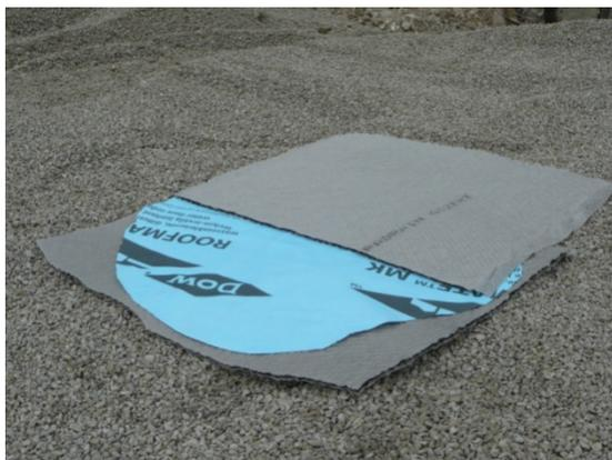
*Protection of heat insulation from rain by watertight liner that is open for water vapour diffusion from down up (blue liner). This liner itself has to be protected from damage by protective geotextiles on both sides of the liner.*
