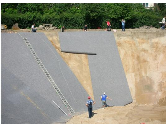
*Protective geotextile is rolled down the pit in lanes*
