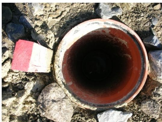
Casting of protection pipe into the borehole. This pipe stays in the borehole and protects the first 5 m depth from weak ground material that could fall in the open borehole.
