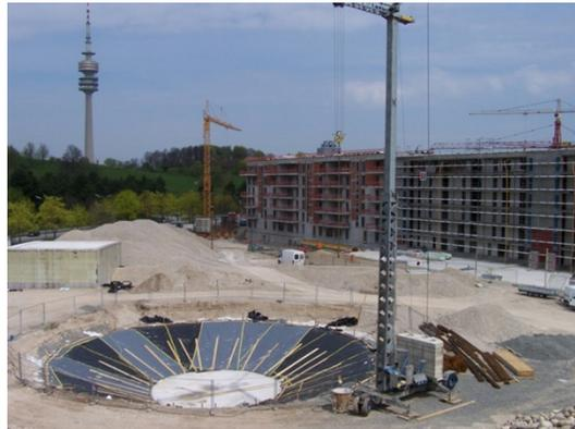
*Concreted bottom plate, watertight liner on geotextile on foam glass gravel*
