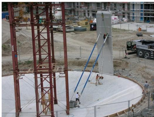
Stabilizing of prefabricated wall elements. Elements are mounted close together.
