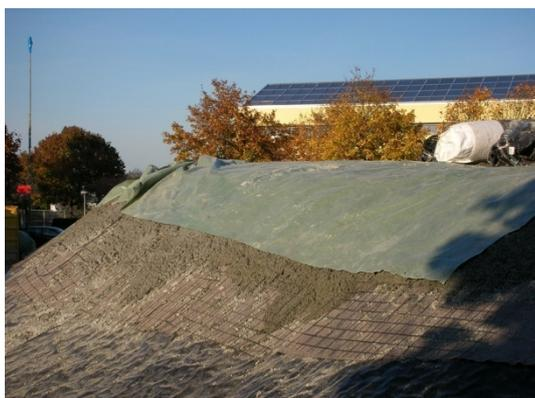
*According to the landscape architecture the outer surface is built up. If the surface of the storage is used by public, a layer of simple concrete to protect the watertight liner from damage is hardly recommended.*
