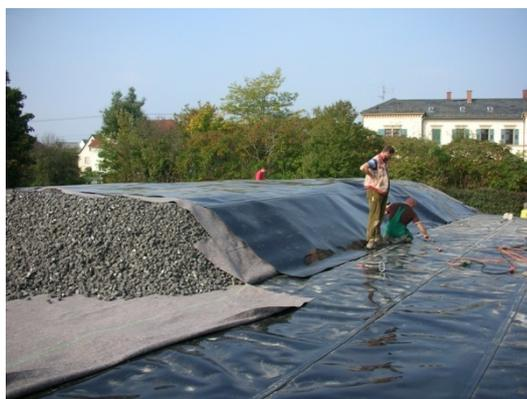
*The upper gravel layer is protected by a geotextile and the inner liner. After the welding from the outside is finished, another geotextile is rolled out for protective measures and heat insulation material (foam glass gravel) is filled up. To prevent the heat insulation from possible rain the process can be parted in daily containment sizes that allow to cover the heat insulation with the outer liner in one day.*
