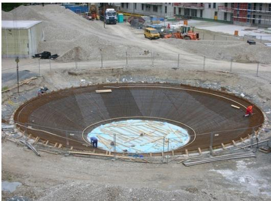
*Reinforcement work on blinding concrete, that was emplaced on watertight liner*
