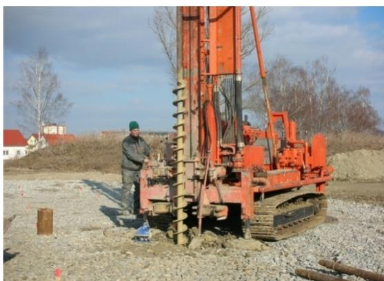
Start of drilling with an auger drill for the first 5 m depths.
