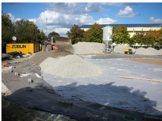
*After the middle sand layer is completed, again a geotextile is rolled out for filling up with the upper gravel layer*
