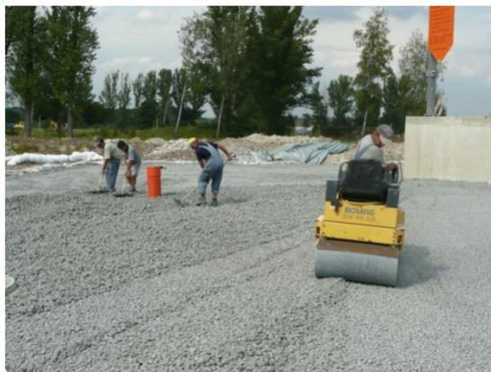
*Preparation of the heat insulation by compacting for covering by liners*
