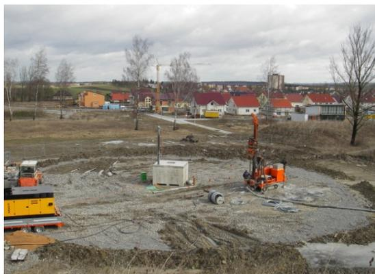
*The drilled out ground is purged to the surface by water pumping. This causes the need for water drainage on the drilling area (photo shows the gravel bed and the drainage ditch round the drilling area)*
