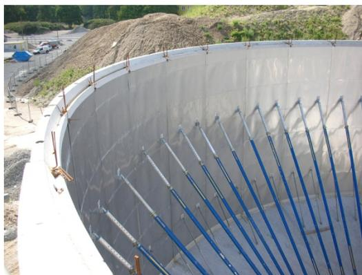
Closing of the cylinder with altogether 26 prefabricated elements, upper part realized as pressure ring.
