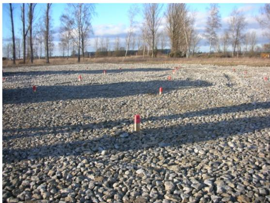
Gravel bed for drilling machine. The positions of the boreholes are determined by measurements and fixed by wooden pegs
