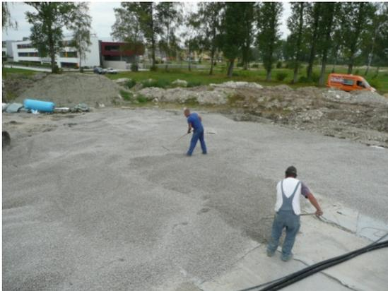
*Leveling of gravel layer for drainage purposes*
