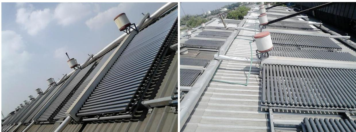
Figure 9: Evacuated tube collectors on the roof of Wheels India in Padi, Chennai, with a collector gross area of 1,365m<sup>2</sup> (Source: IEA SHC Task49 & SoPro India)
