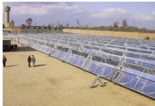
Fig. 12: Solar thermal process plant - steam production in chemical industry (source: Fichtner Solar GmbH, Germany)
