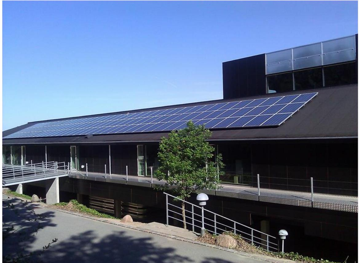
*86 m<sup>2</sup> heat collector mainly for hot water (production 3 kWh/m<sup>2</sup> heated floor area per year)*
