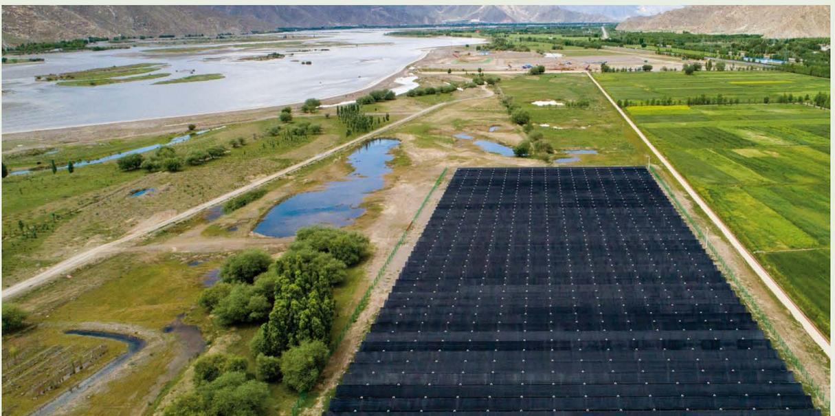
Lasha solar district heating system in Tibet, China with  $13,000 \text{ m}^2$  collector area ( $9.1 \text{ MW}_{\text{th}}$ ). Photo: Solareast Holding Company Ltd.
