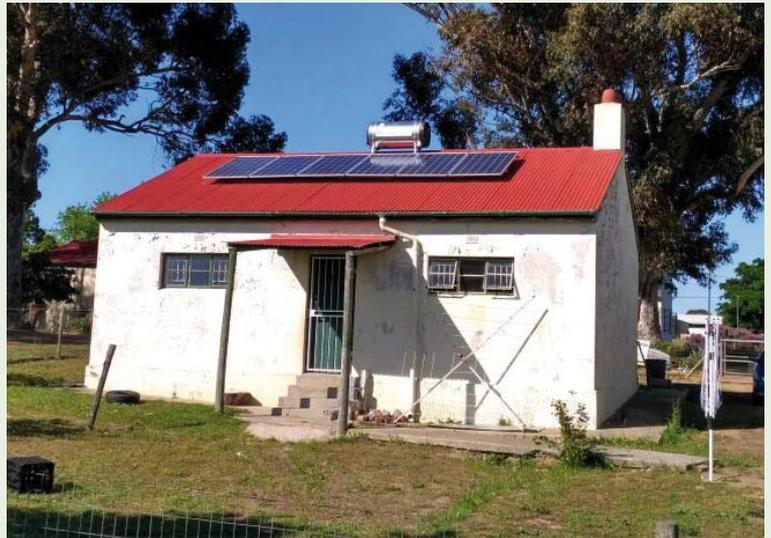
*PV2heat system at the Mariendal Experimental Farm of Stellenbosch University in South Africa consisting of 1.5 kW<sub>peak</sub> PV and a 200-liter hot water tank.*
