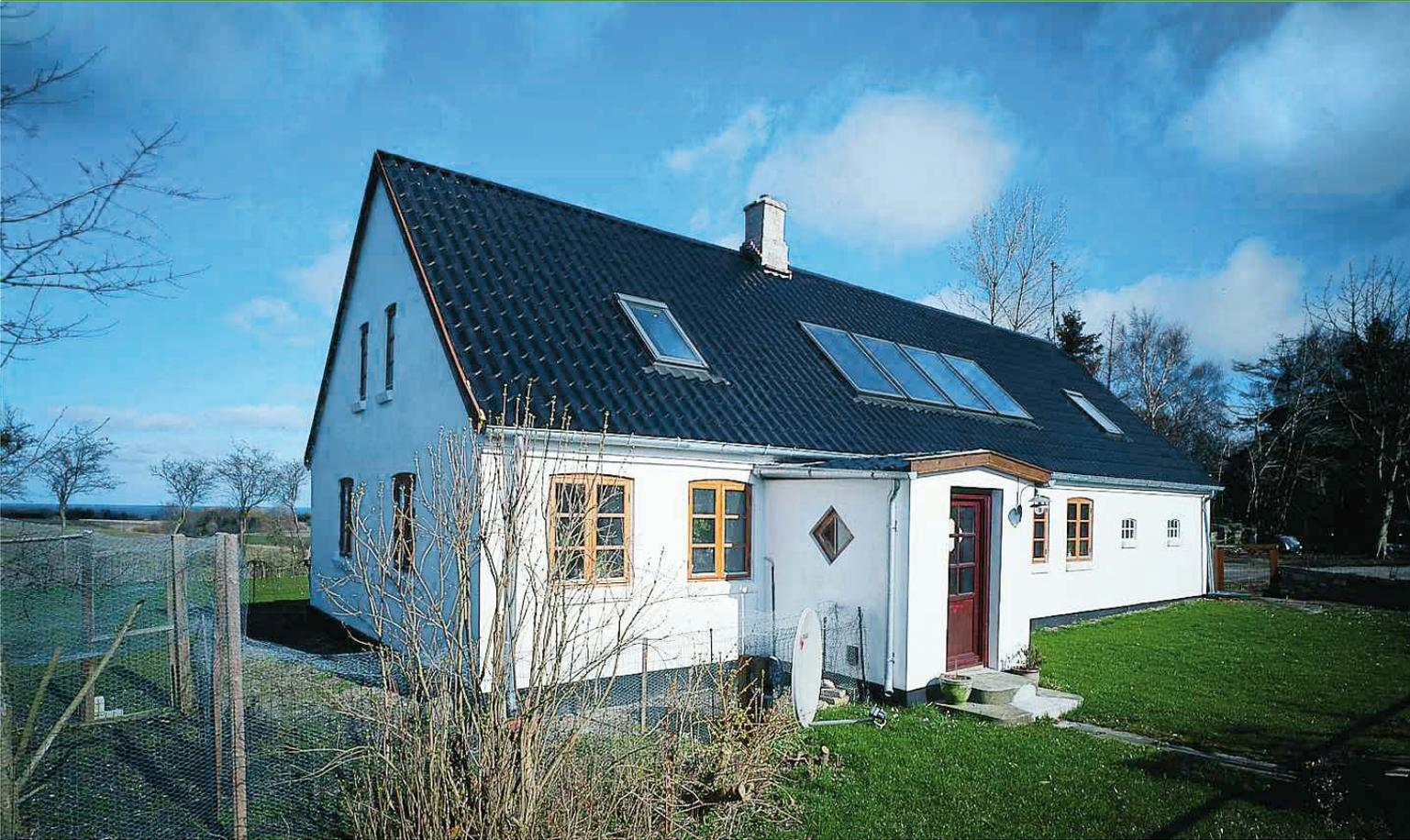
Typical pumped solar thermal system for water heating for a single-family house.
