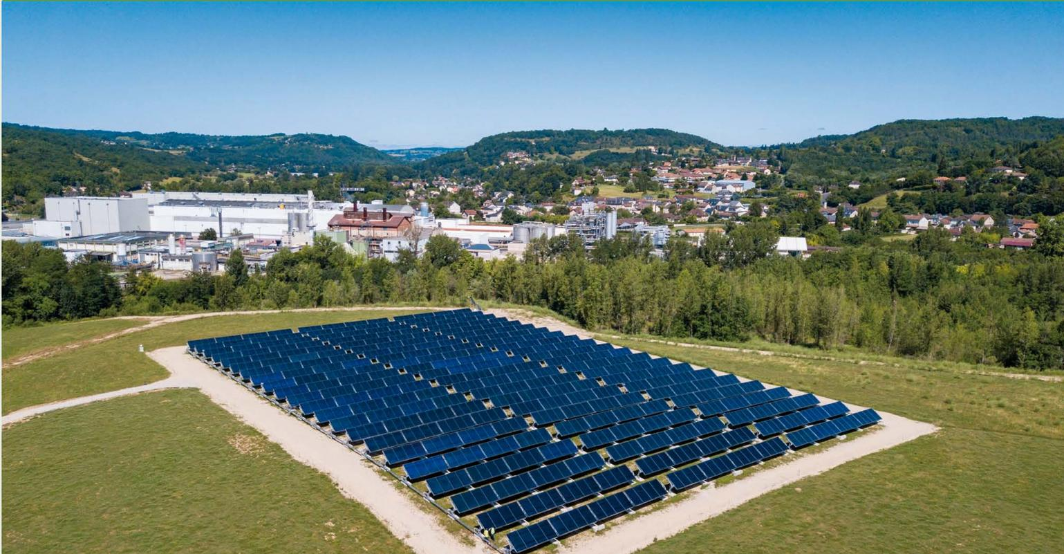
2.9 MW<sub>th</sub> flat plate collectors on trackers provide heat for the CONDAT Paper Mill in France
