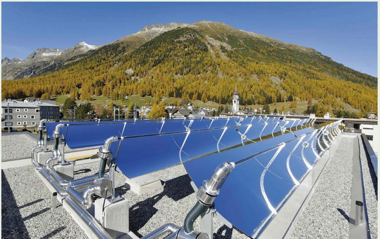
*Lataria-Engiadinaisa-Dairy, Switzerland with 115 m<sup>2</sup> of parabolic trough collectors*
