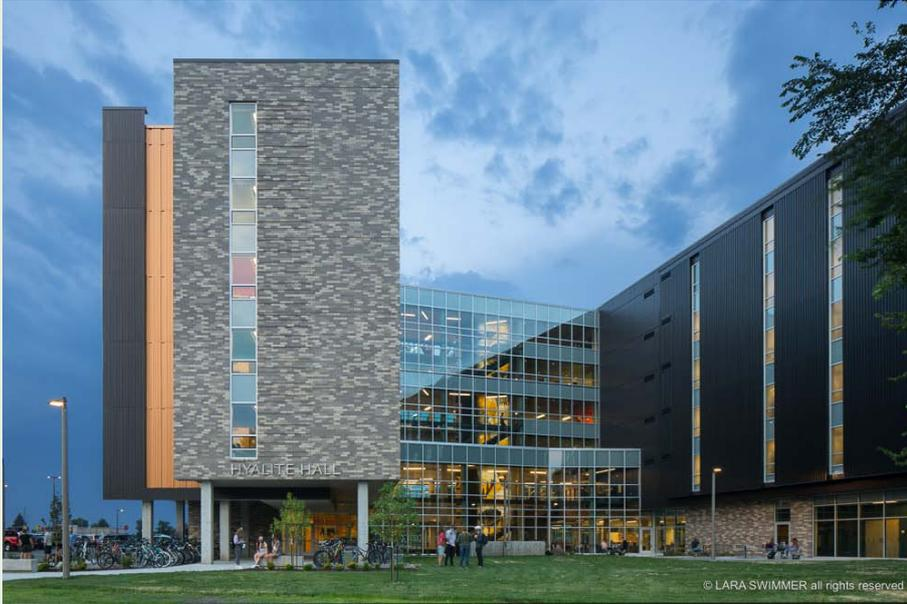
0.6 MW<sub>th</sub> façade integrated solar air system at Hyalite Hall, Montana State University, Bozeman, USA.
