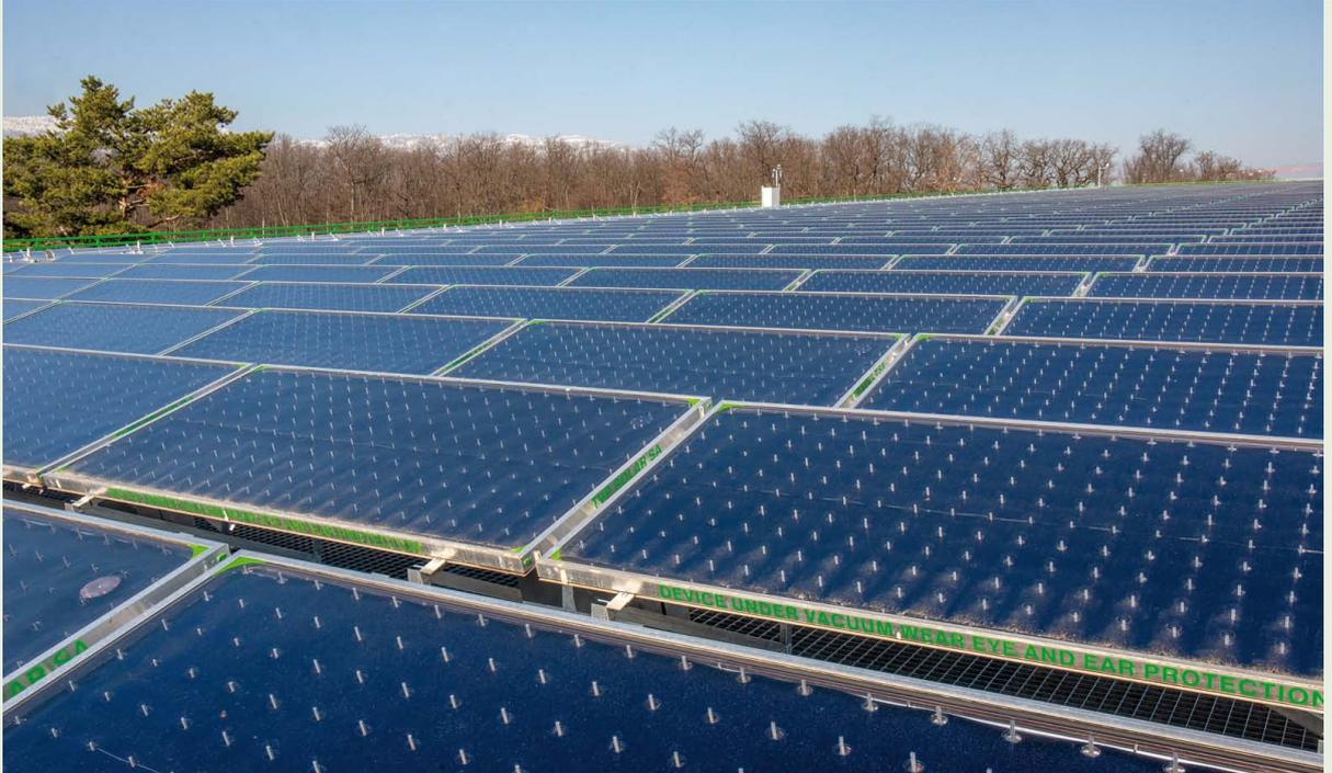
The Swiss solar district heating system in Geneva, with a capacity of  $0.5 \text{ MW}_{\text{th}}$ , is equipped with high-vacuum flat plate collectors and began operation in December 2020.
