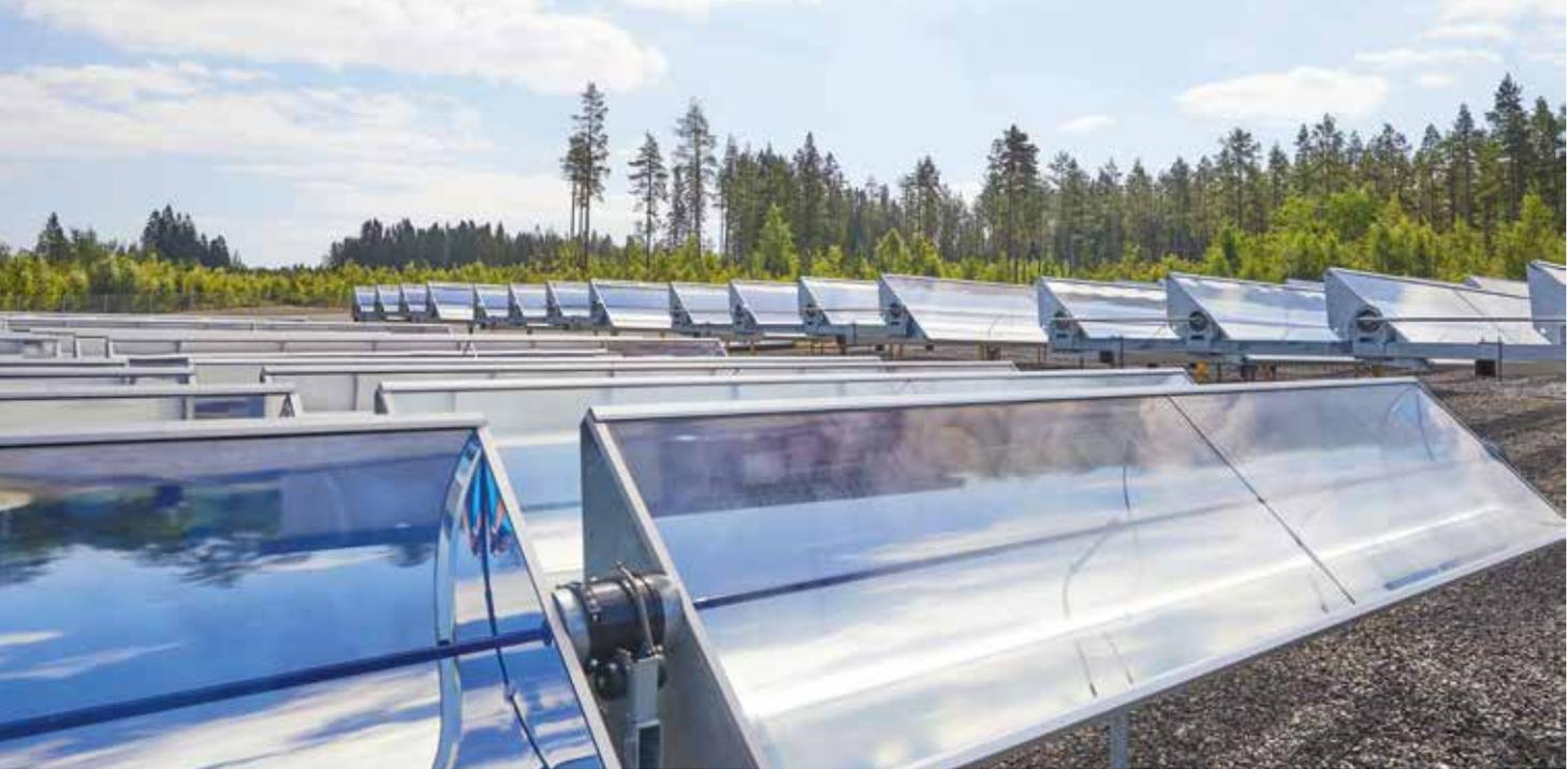
Höglätten solar district heating park with 3,000 m<sup>2</sup> parabolic trough collectors, Sweden
