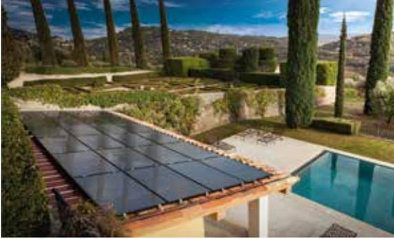
**PVT system with a thermal capacity of 19,1kW<sub>th</sub> and 6kW<sub>peak</sub> on a pool house in Grasse, France**
