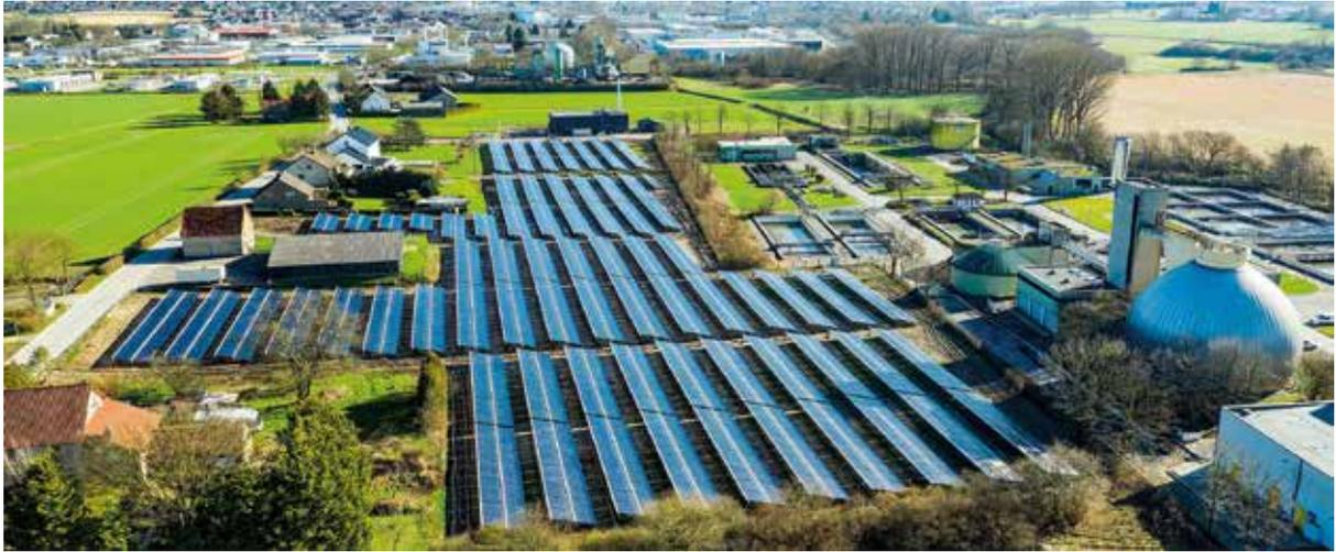
**Solar district heating plant in Lemgo, Germany, consists of 9,181 m<sup>2</sup> vacuum tube collectors**
