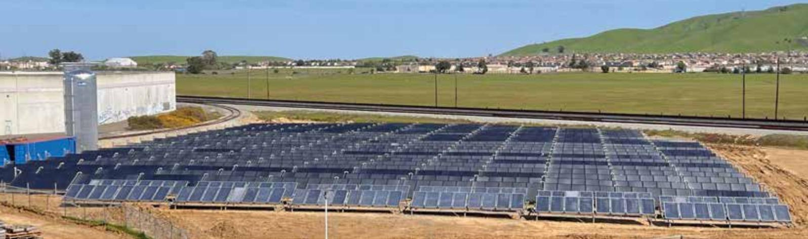
**Solar process heat system at the Ball Corporation, headquartered in Fairfield, California, USA. Flat plate collectors with a capacity of 2.8 MW<sub>th</sub> (3,956 m<sup>2</sup>) provide the heat for washing beverage aluminum cans**
