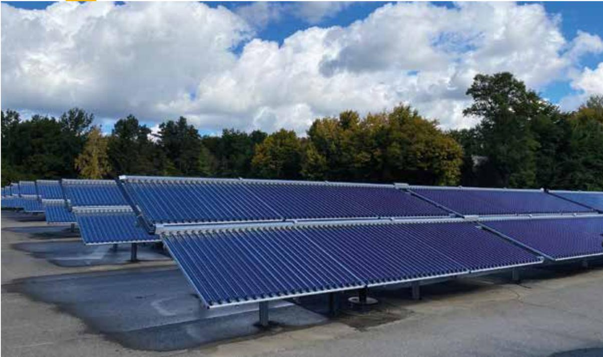
**Solar district heating Sigmaringen in Germany with 2,312 m<sup>2</sup> collector area in connection with a 400 m<sup>3</sup> heat storage**
