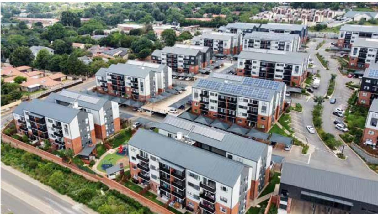
**14<sup>th</sup> Avenue housing project in Johannesburg, South Africa. The project consists of 15 solar thermal systems with a total collector area of 531 m<sup>2</sup>**
