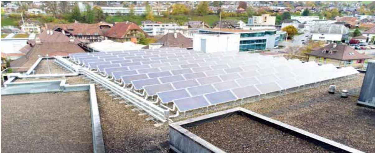
A leading Swiss milk processing company uses 147 kW<sub>th</sub> (210 m<sup>2</sup>) of high vacuum flat plate collectors for cheese production
