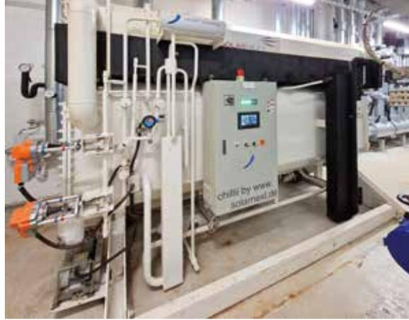
**Solar thermally driven 348 kW cooling capacity water/LiBr absorption chiller for air-conditioning at 16/10 °C chilled water temperature in Mali**
