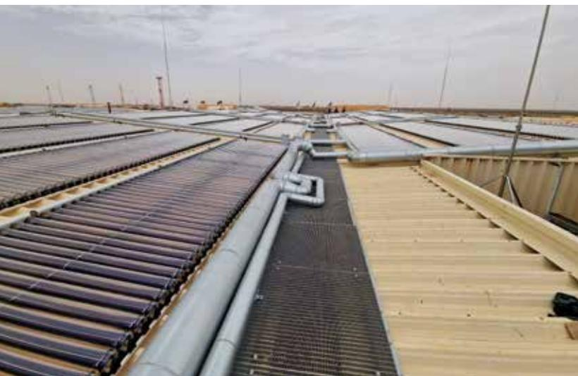
**700 m<sup>2</sup> vacuum tube solar collectors supply heat to drive a 348 kW water/LiBr absorption chiller for air-conditioning a new cafeteria and kitchen at Camp Castor in Mali**
