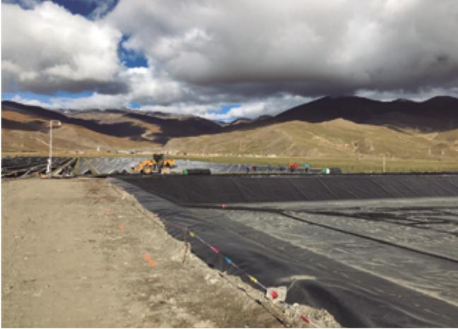
2. Add a watertight liner at the bottom of the pit.
