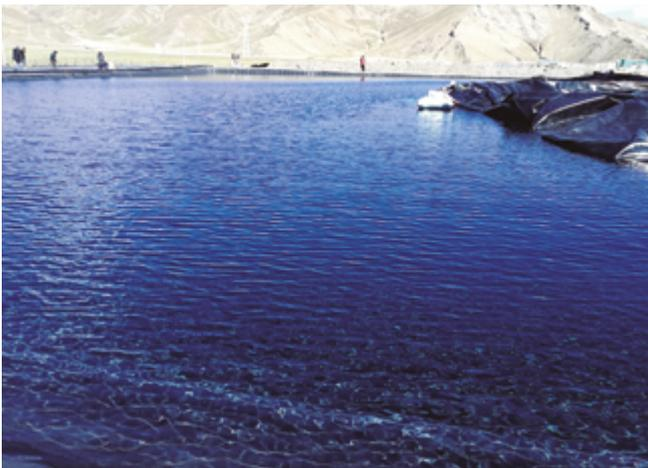
4. Put an insulating and floating cover on top.
