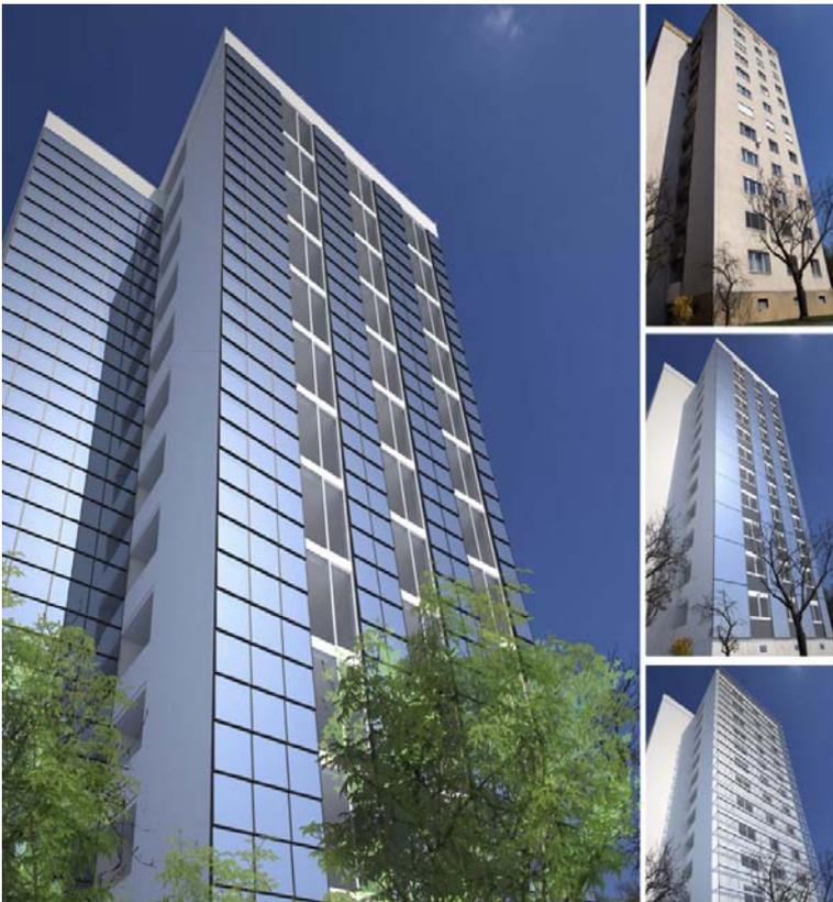
Figure 6: Alternative approaches for integrating solar thermal collectors into high rise apartment building from the late 1960 in the course of a renovation study, Source: Institute of Architectural Typologies, Graz Technical University
