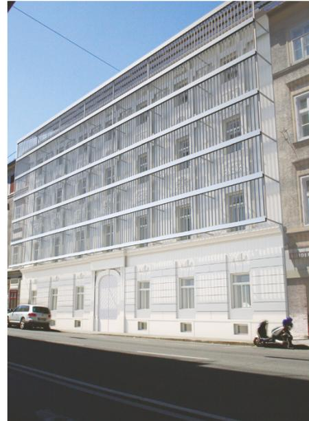
Figure 4: Visualization of proposal for evacuated tube collectors in front of listed building façade in Graz, Austria. Source: Institute of Architectural Typologies, Graz Technical University
