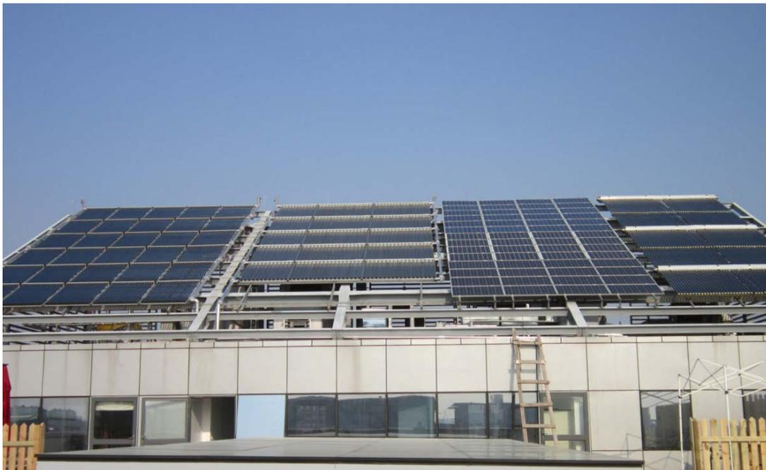
**Figure 25: Installation of vacuum tube collectors (heat pipe + CPC), PV panels and solar air collectors at the GEL building from the left to right (Source: SJTU)**
