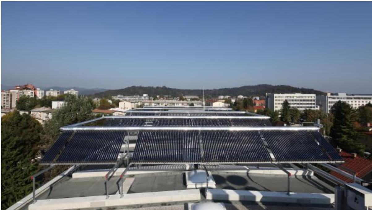
Figure 13: Vacuum solar collectors on the roof of the Jožef Stefan Institute (Source: JSI)
