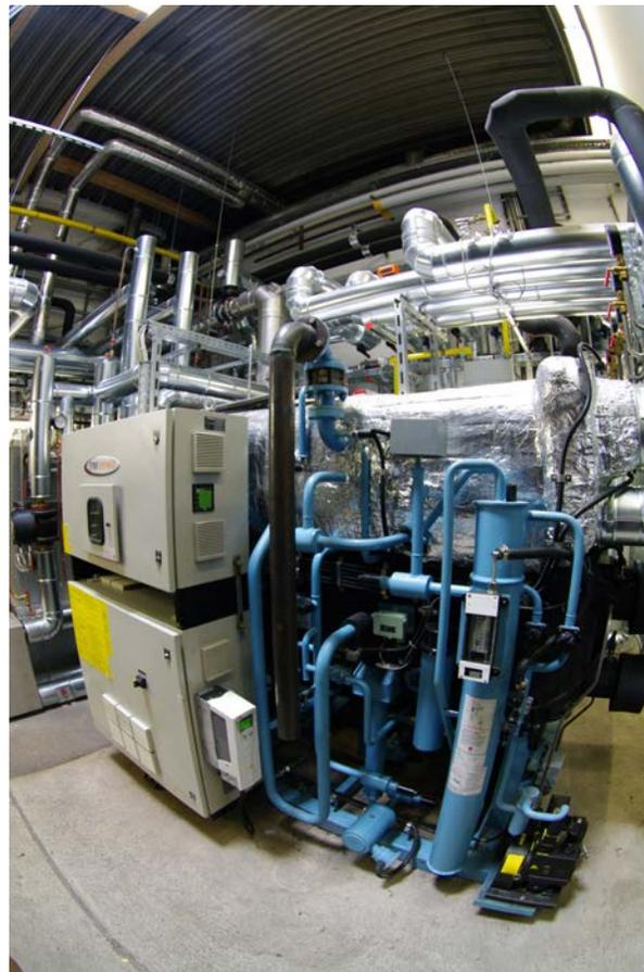
Figure 9: Solar/gas driven single-/double-effect absorption chiller at Lindner (Source: ZAE Bayern)
