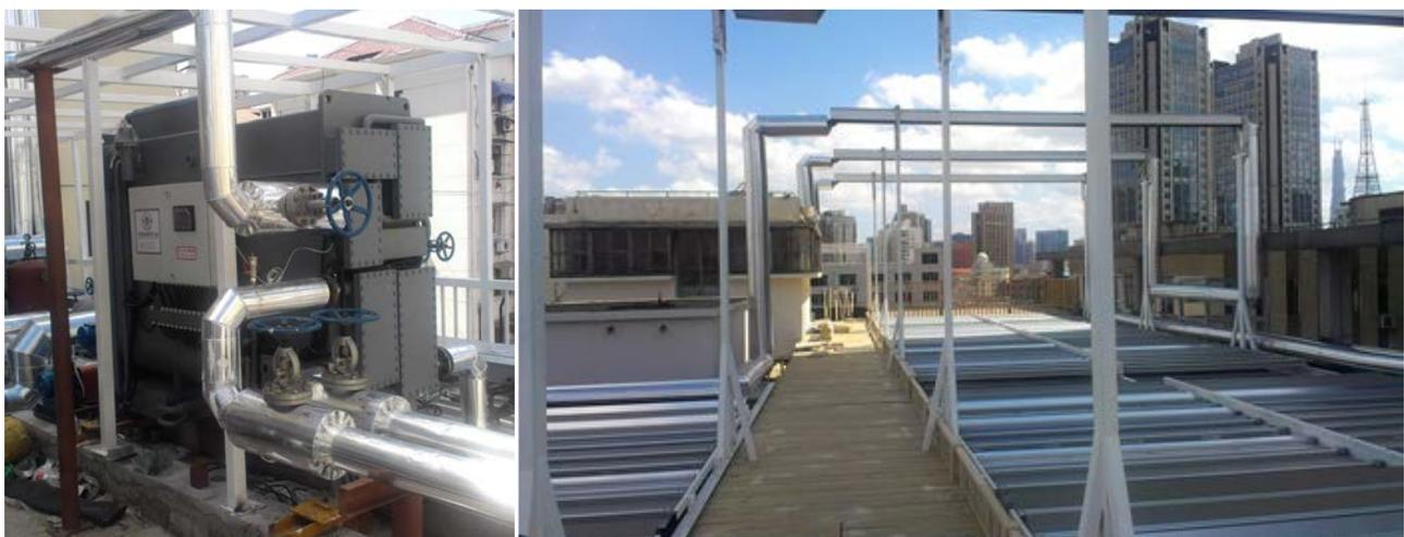
**Figure 22: Single-/double-effect absorption chiller and Fresnel collectors on the roof of the Shanghai Electric office building (Source: SJTU)**
