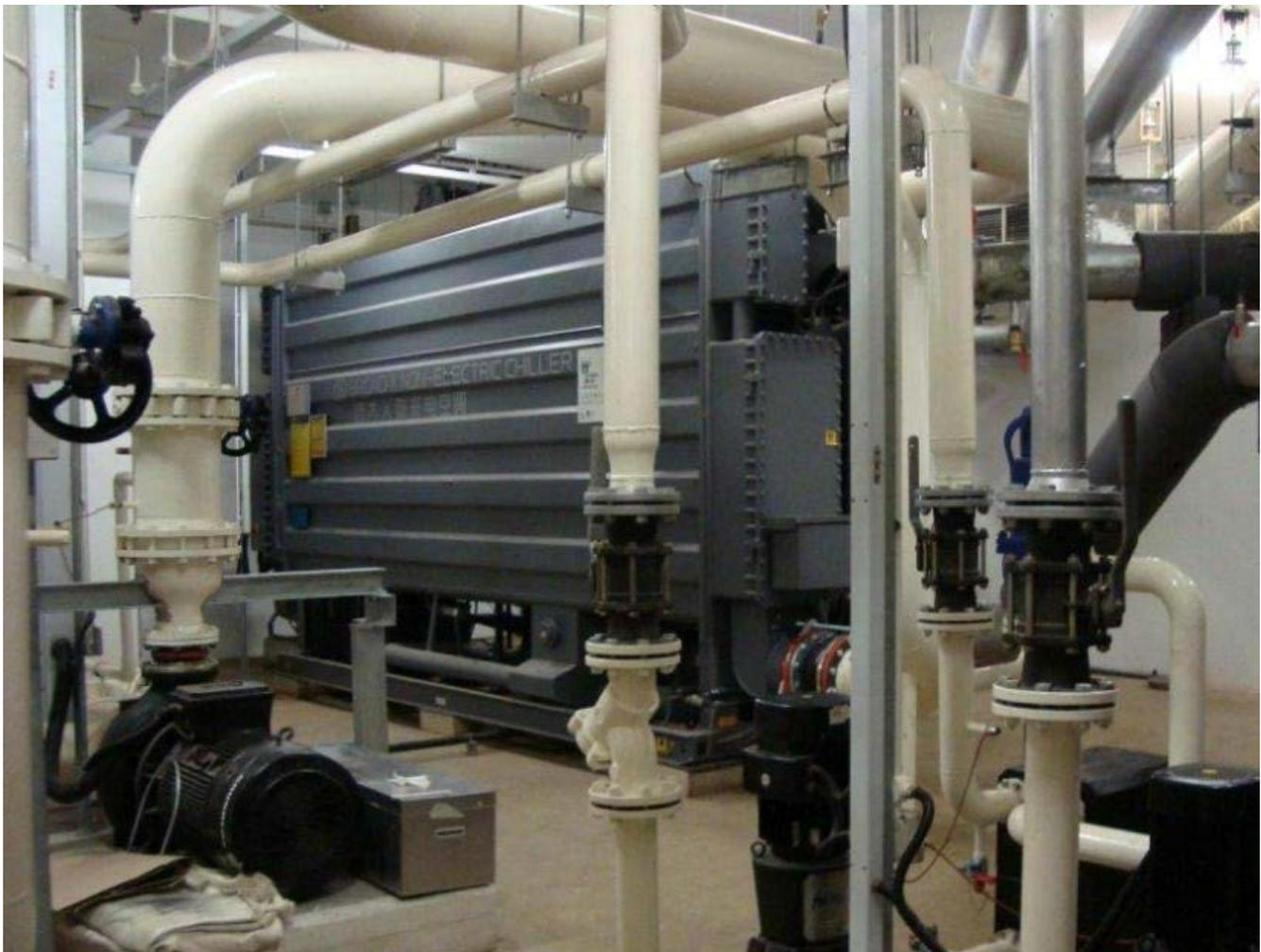
Figure 3: Absorption chiller with 1,750 kW cooling capacity (Source: SOLID)
