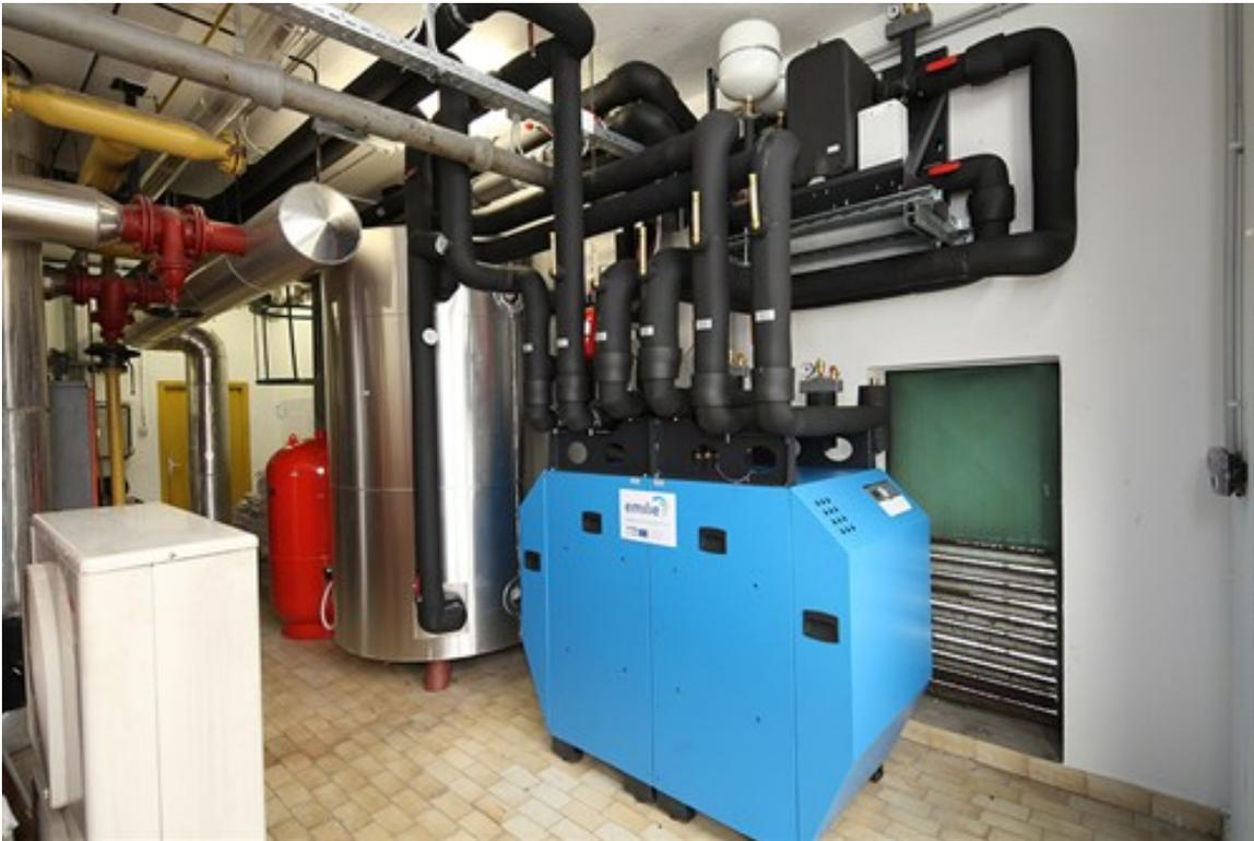
**Figure 14: Installation with 20 kW adsorption chillers and heat storage (JSI)**
