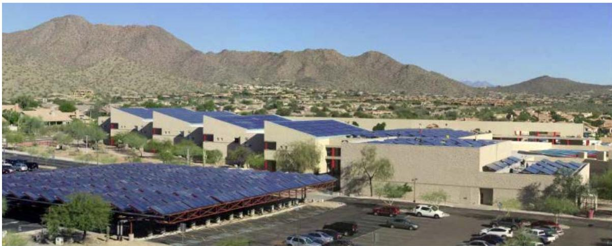
Figure 2: Roof mounted solar collectors at Desert Mountain High School (Source: SOLID)
