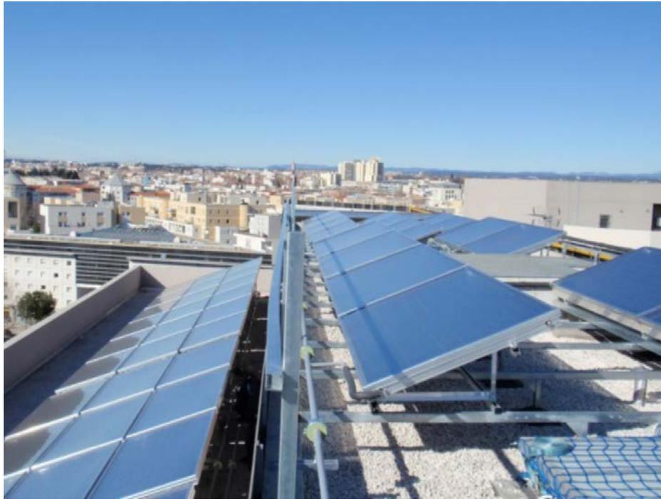
Figure 5: Solar collector fields with drain back system (Source: TECSOL)
