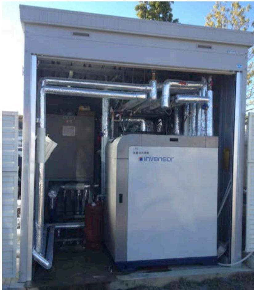
Figure 28: Adsorption chiller of the solar cooling system (Source: InvenSor)
