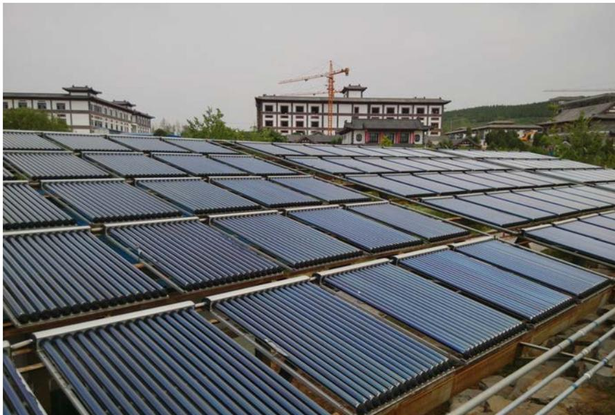
Figure 18: Installation of evacuated tube collectors on the roof (Source: SJTU)
