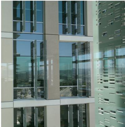
Figure 5. Exterior vertical fins on east and west facades.
