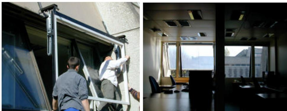
Fig. 13 Real 1:1 scale experiment within the TwinCells (right). Left Room is equipped with tiltable Serraglaze window (left).
