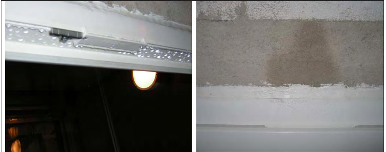
Figure 5.8: Condensation in the window frame, ventilation opening and wetting of the wall at the top side.
