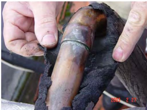
c) Inexistent mechanical protection for insulation
