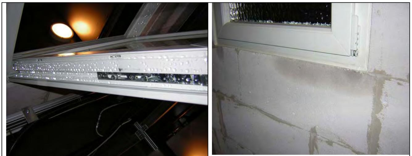
Figure 5.7: Condensation in the window frame and wetting of the wall at the bottom side.
