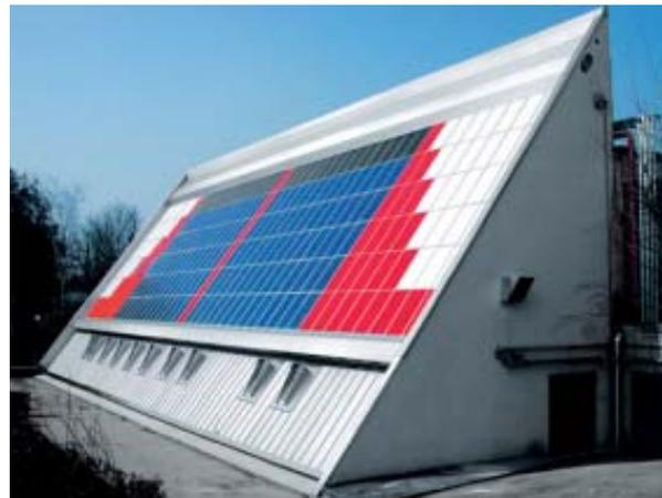
Figure 4: Ventilated PV with heat recovery – TIS from Secco Sistemi mounted on Centro Ricerche Fiat di Orbassano, Torino, Italy.
