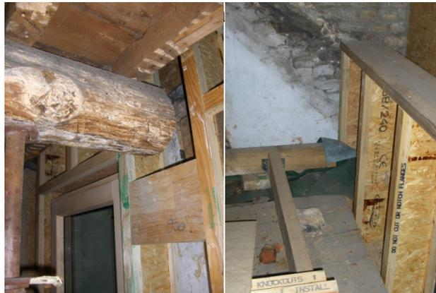
The I-beam construction cutting through the floor slab and support beam (left) and ending above the upper floor level, next to the new roof construction (right). The brick wall clearly shows where the old roof was.
