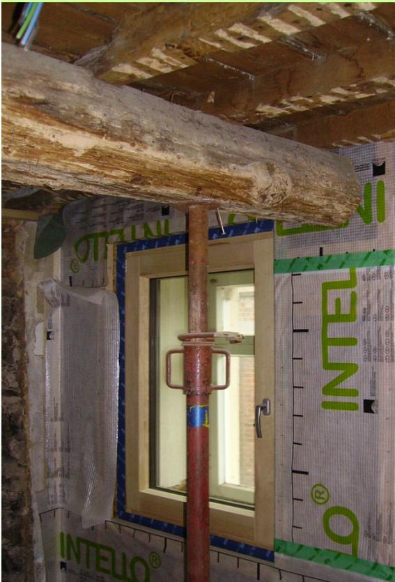
Problem of air tightness on old beam. Note the 'intelligent' air and vapour tightness screen. The screen's vapor resistance is varying depending on the relative humidity, going from 0.25m to 10.5m.
