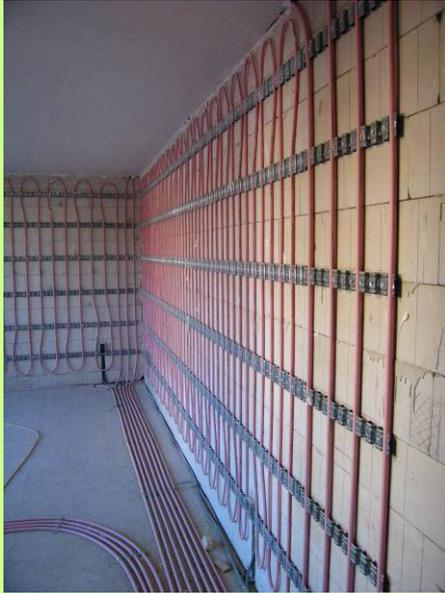
Silicate block wall and surface heating tubing.
