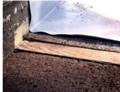
Detail of the EPDM liner over the cork insulation
