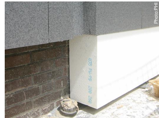
Plinth insulation without an end profil. The downpipe is conducted through a cavity in the insulation. The thermal bridge ( $\psi_a = 0.025 \text{ W/(mK)}$ ) is acceptable if the remaining insulation is at least 100 mm.
