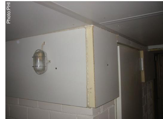
Flanking insulation of the interior wall in the basement with polyurethane boards of 40 mm.
