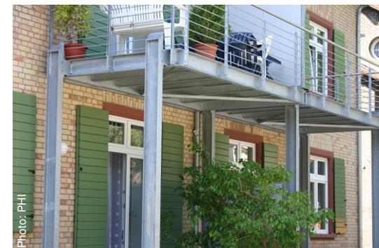
Reduction of thermal bridges by constructing new stand-alone balconies.
