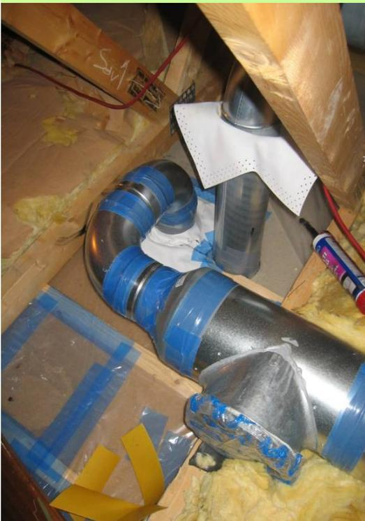
Sleeves (white) are used for tightening between the vapour barrier and the ventilation ducts penetrating the attic floor before insulation is added. (The sleeve to the right is not mounted yet)
