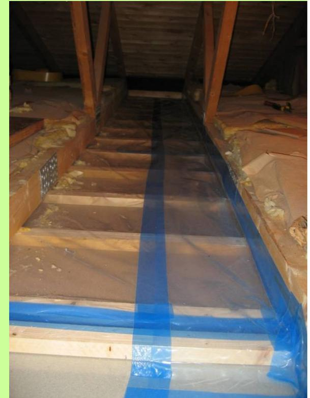
Tightening of the vapour barrier towards the attic
