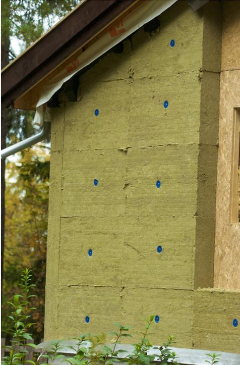
A layer of studs / OSB panels outside the old log walls were needed to achieve an even surface for the facade insulation, which was anchored to the OSB with long screws..
