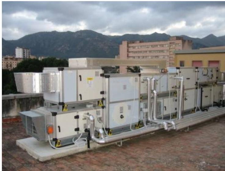
Air handling unit desiccant cooling (AHU-DEC)
